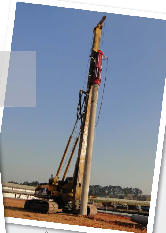
Cravamento de Ø 500 mm / Driving piles up to Ø 20 in
